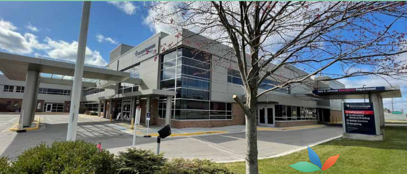
The updated Dale E. Johnson Emergency Department at OMH features separate entrances for patients and EMS, which streamlines traffic for staff, patients, and visitors.
